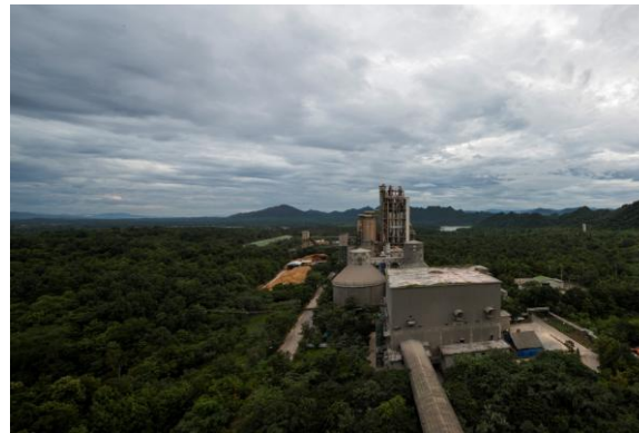
All cement plant
