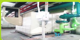
Fresh Air Supply 10 cfm/man - 5M baht
