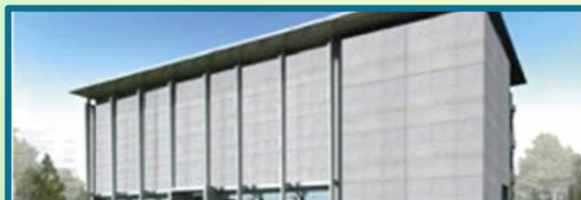
Data Center Park High-Quality Infrastructure Flood Protection
