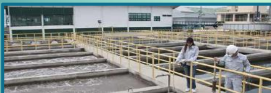
Waste Water Treatment Plant 4 Plants : 50,500 m3
