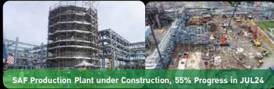
SAF Production Plant under Construction, 55% Progress in JUL24
