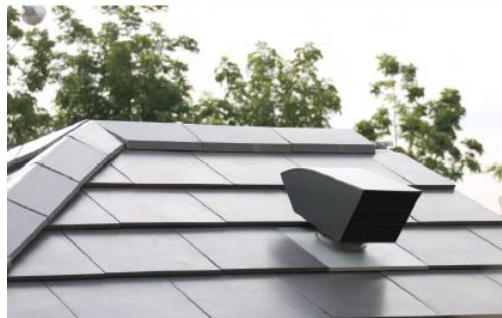
Example of a Passive Ventilation System, which cools the Attics with natural wind at Noble Gable Watcharapol Project
