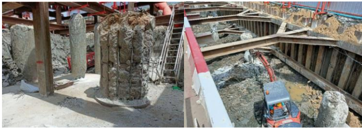
Pile Cut Off to for Recycle
